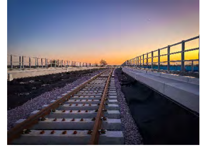
New track on Bletchley Flyover, January 2022
